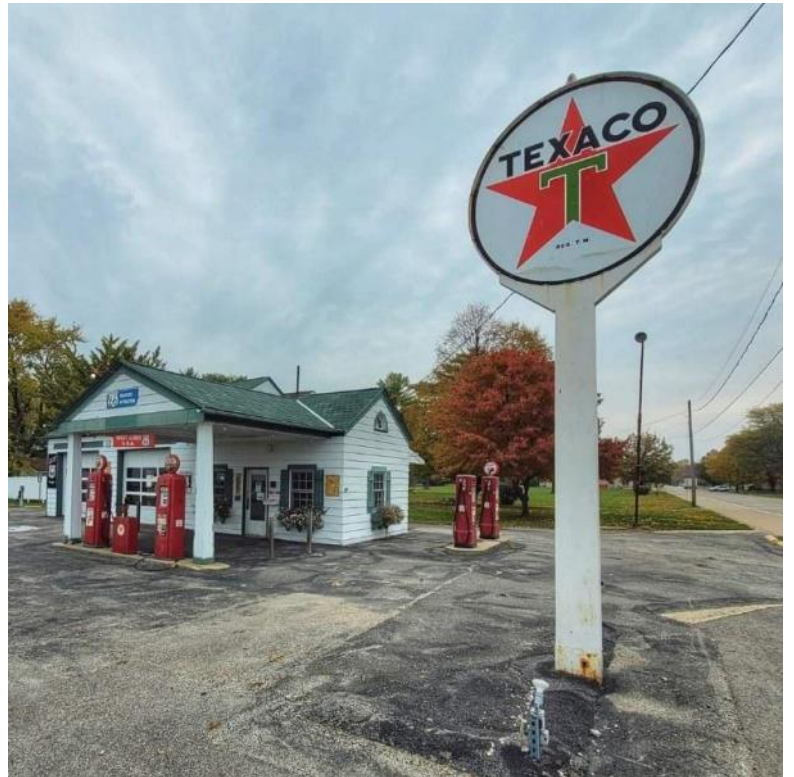
Restored Texaco station on Route 6 in Dwight, IL. -John Brewer
